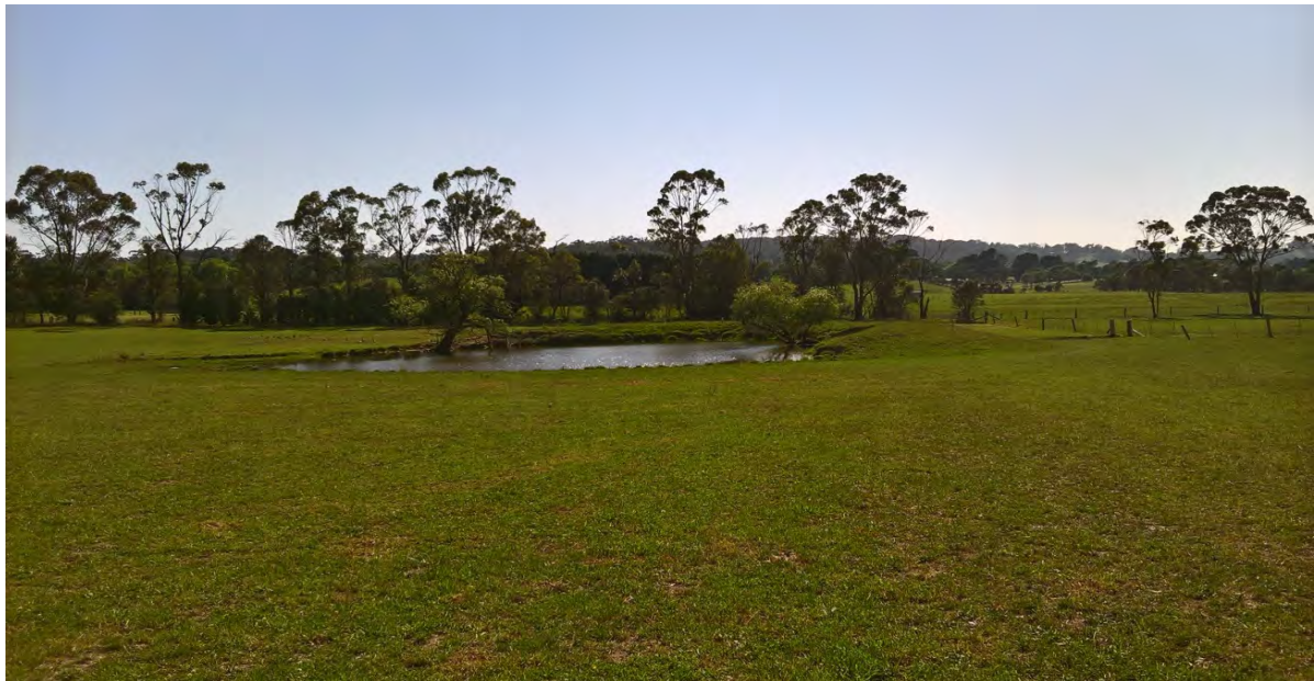
Photo 5: View of dam and dam embankment.
