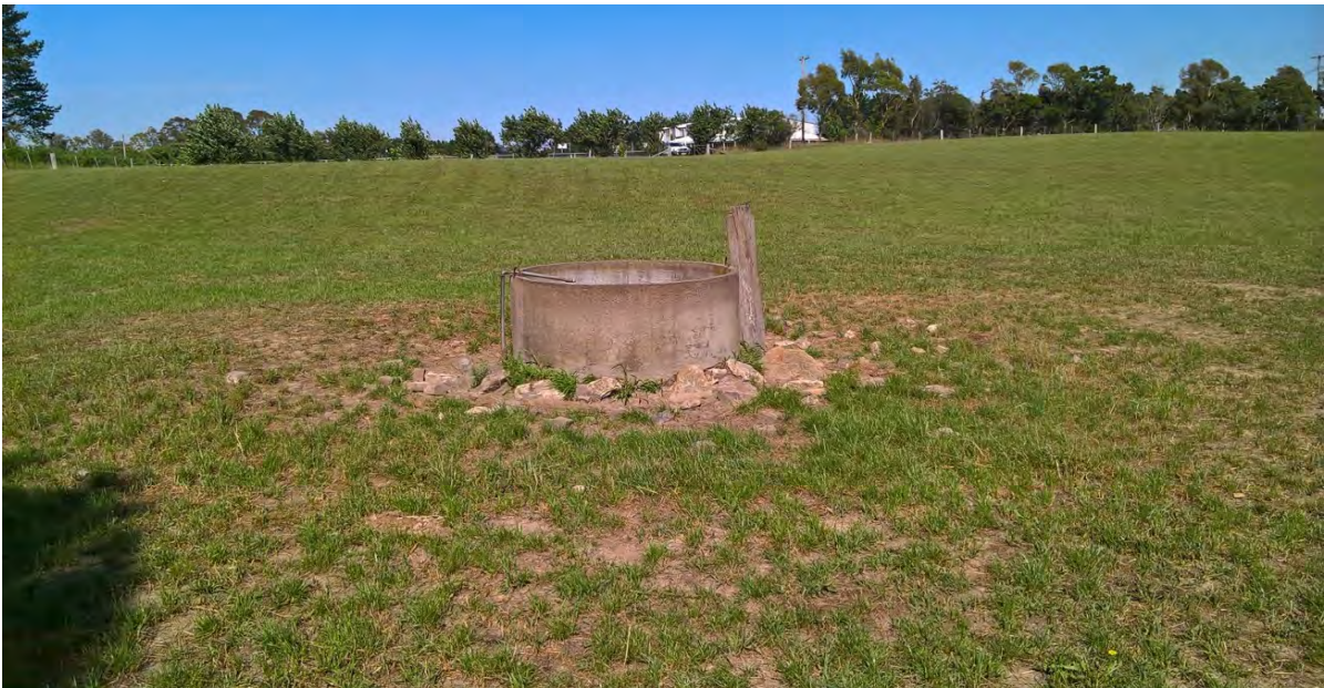
Photo 3: View of water trough with brick and concrete at the base observed in the southern central portion of the site.
