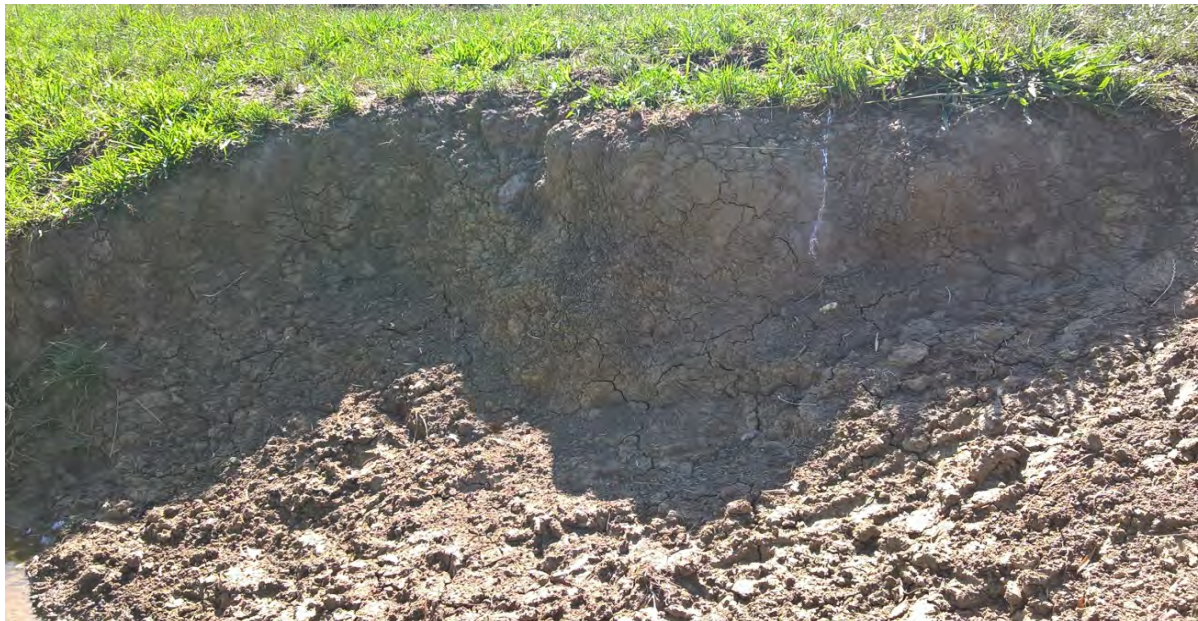
Photo 6: View of exposed soils in dam embankment.
